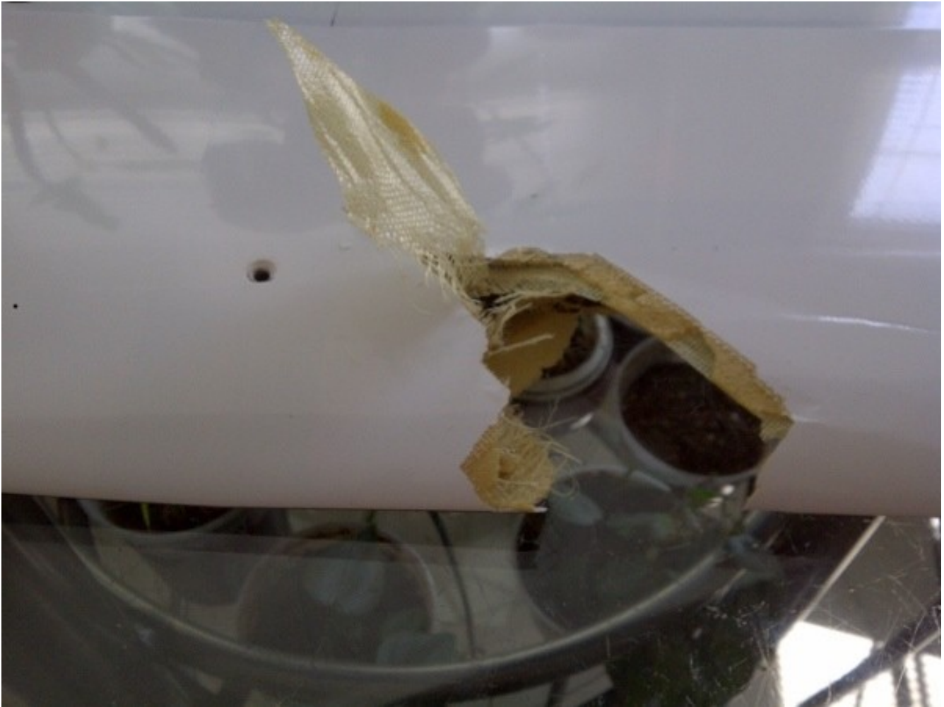
Removing damaged material. Look closely and you can see how coarse the Kevlar netting is and the creases in the wing.
